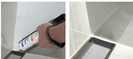
To cover the visible edge of the PVC channel, use a fine sandpaper to rough the channel's top edge. Use a bead of a epoxy based silicone that is similar in color to the finishing grout **OR** Use a 1:1 mixture of clear PVC cement and desired dry unsanded grout, and apply immediately along the visible edge. Clear PVC primer solvent should be used on the channel edges before applying PVC/grout mix.
